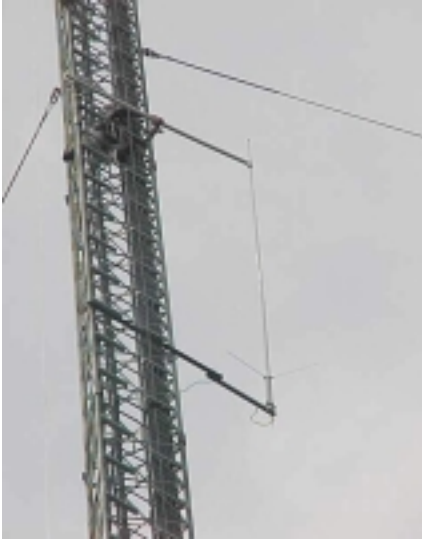
N5AGG on the tower fitting the top support bracket on the antenna
