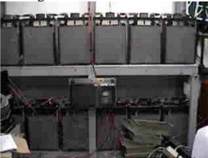
24-volt battery bank with wind generator controller
