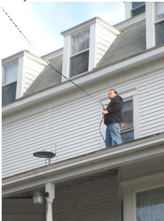
Steve and Bruce then checked the antenna's ability to be tuned by my MFJ KW antenna tuner and everything was a go. All the bands could be tuned to less than 1.5:1 SWR.
