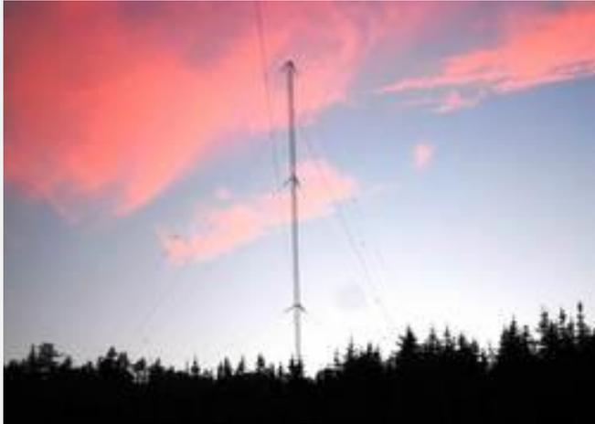
*VO1NA says this tower serves as a monopole antenna for 2200, 1600, 600, 160, 80 and 60 meters and holds up the far end of a wire that also is used on these bands.*
