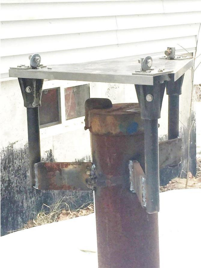
Needless to say that that foundation footing is not going to move. Also the well casing should provide an additional grounding point for the hefty vertical.
